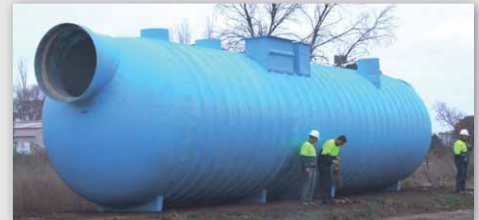
SPEL STORMCEPTOR™ CLASS 1 on site ready to be installed, as part of a treatment train in a Water Sensitive Design project for the Penrith City Council at Lambridge Estate and Penrith Lakes NSW.
