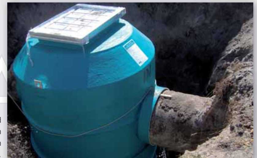
SPEL STORMCEPTOR™ CLASS 1 on site ready to be installed, as part of a treatment train in a Water Sensitive Design project for the Penrith City Council at Lambridge Estate and Penrith Lakes NSW.
