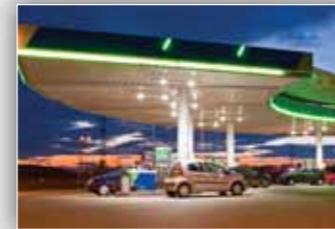
Service Stations & Refuelling Zones
